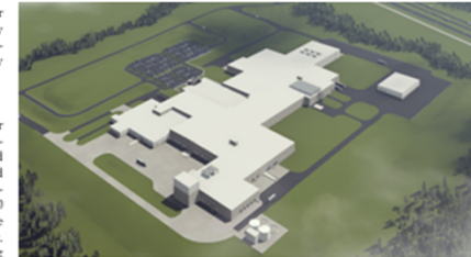
American Foods Group is building a new $800 million beef processing facility in Warren County, Missouri.
