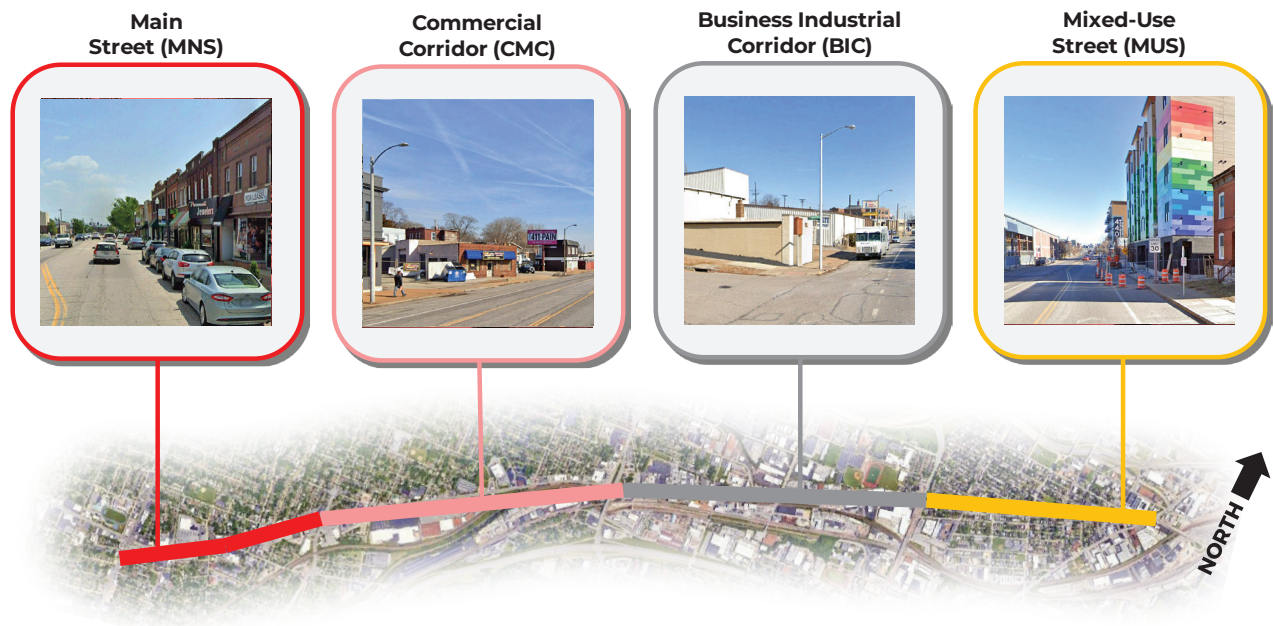
FIGURE 1-32: Manchester Road / Route 100 Context Example in the City of St. Louis and St. Louis County
