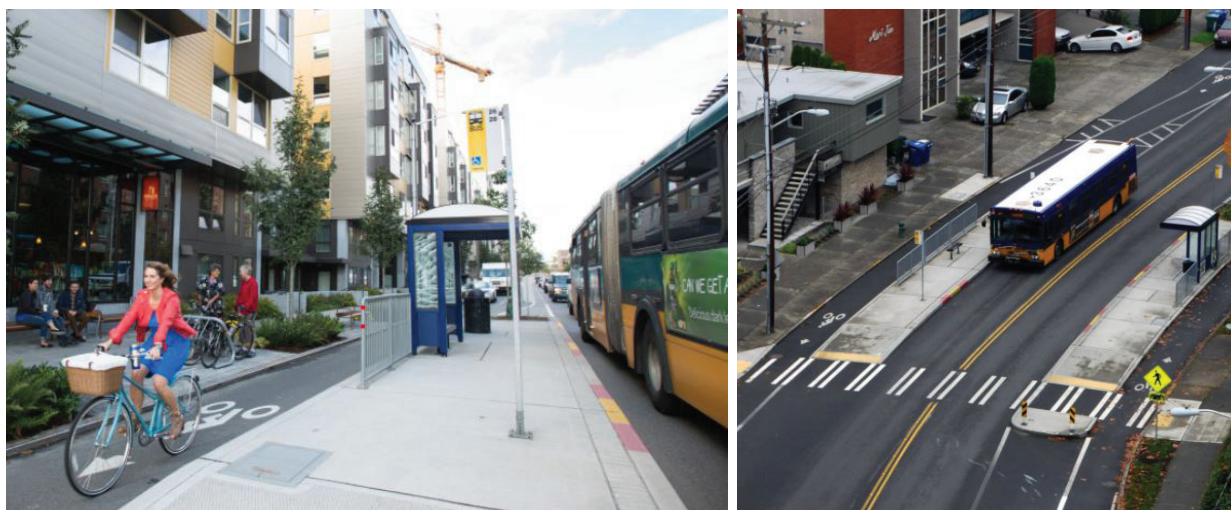
Examples of Mobility Hubs and Floating Transit Islands courtesy of NACTO Transit Street Design Guide
