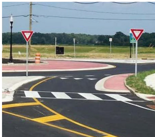
Example of a truck aprons that reduce turning radii for vehicles in Ohio and New Jersey, courtesy of FHWA Achieving Multimodal Networks Guide
