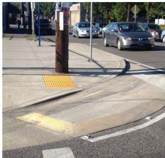
Example of a truck aprons that reduce turning radii for vehicles in Ohio and New Jersey, courtesy of FHWA Achieving Multimodal Networks Guide
