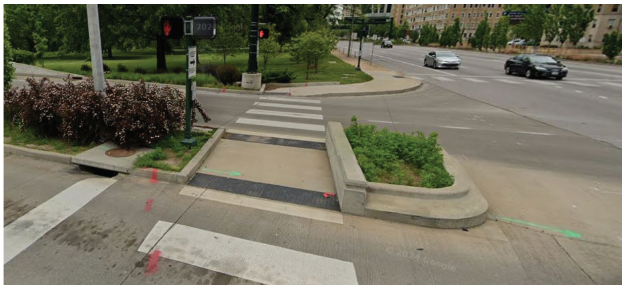
Example of a Pedestrian Refuge Island at Kingshighway and Forest Park Parkway
