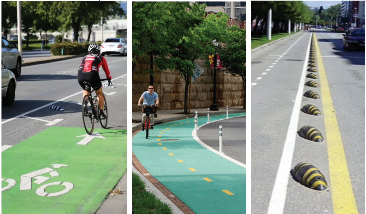
Examples of Dedicated Bike Lanes (Green, buffered, protected, etc.) courtesy of NACTO Bike Design Guide and recycled armadillo dividers courtesy of Inhabit
