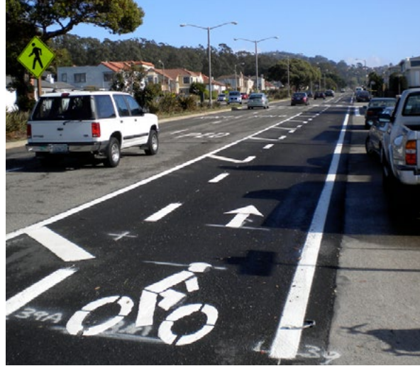
The use of pavement markings delineates space for cyclists to ride in a comfortable facility.
