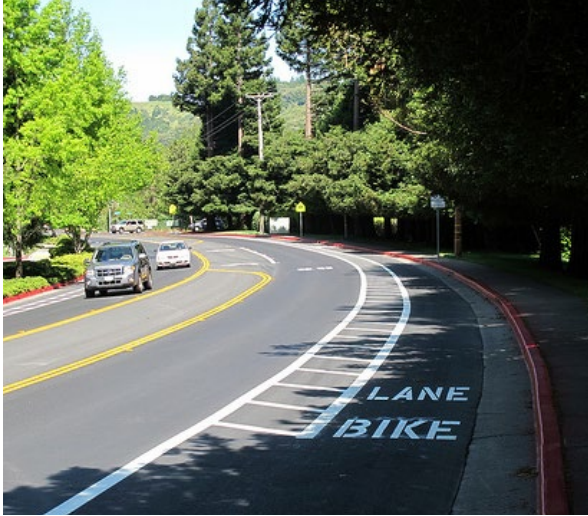
The use of pavement markings delineates space for cyclists to ride in a comfortable facility.
