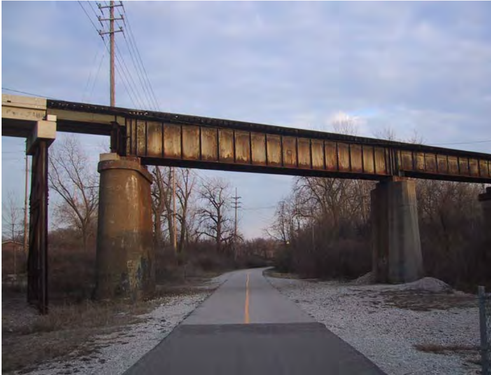
Figure 7-2: BNSF bridge over Grant's Trail near Green Park.
