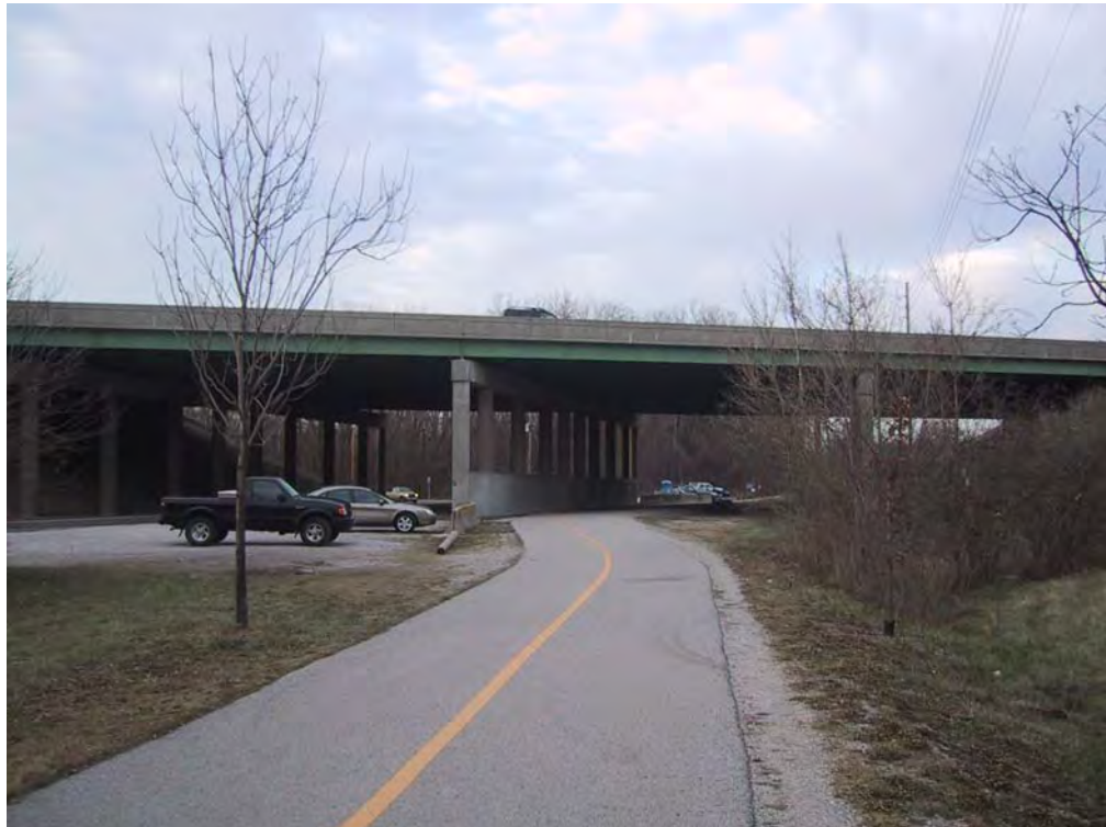
Figure 7-3: Grant's Trail passing under I-55 at Greenpark Road
