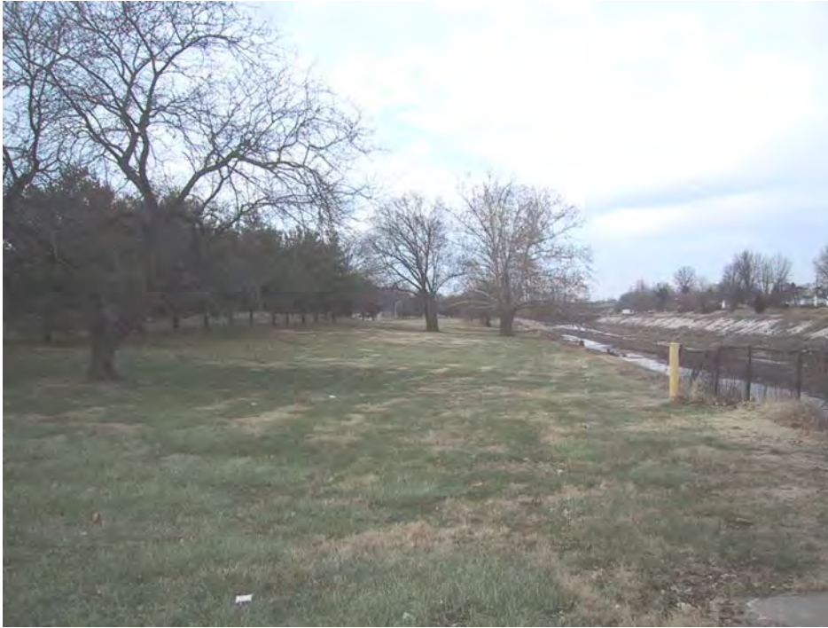
Figure 7-1: River Des Peres Park and Drainage Channel
