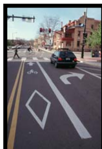
Left: Bicycle lane before and after intersection. Center: Left turn bicycle lane. Right: Bicycle signal actuation. Note: Diamonds are no longer in adherence to accepted striping standards.
