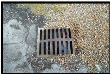
Above Left: An inlet grate can be a hazard for bicyclists especially if the openings are parallel to the direction of travel. Above Middle: Uneven pavements are often located at the edge of two types of pavement, in this case asphalt pavement and a concrete curb and gutter. Above Right: Although a shoulder exists, gravel and other debris may cause it to be unsuitable for bicyclists.
