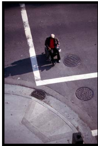
Top Right: Two ADA ramps, one for each direction of travel, are preferred. Bottom Right: Single ramps often force pedestrians into conflict with vehicles to order to access the ramp.
