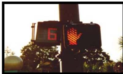
Top Left: Bicycle and pedestrian actuated signal. Bottom Left: Pedestrian actuated signal with “countdown” feature. Right: Pedestrian actuated signal
