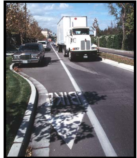
Above: Although there is a dedicated bicycle lane, the presence of the semi-tractor trailer creates an uncomfortable and potentially unsafe bicycling condition. Note: the bicycle lane symbol shown is not in adherence with current standards.
